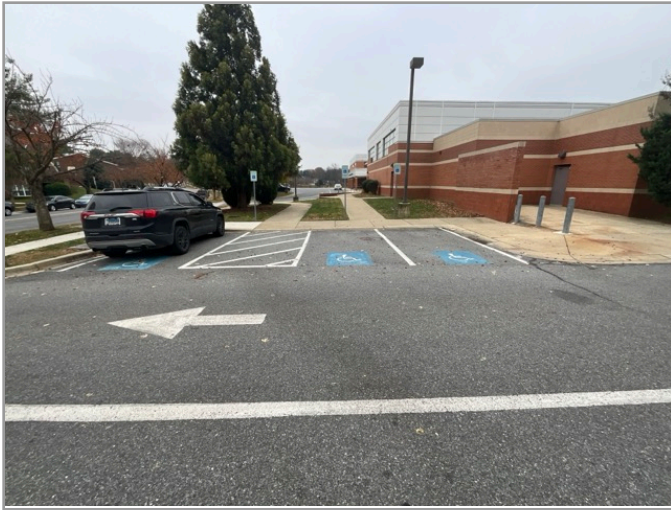
OVERVIEW OF ACCESSIBLE PARKING AREA
