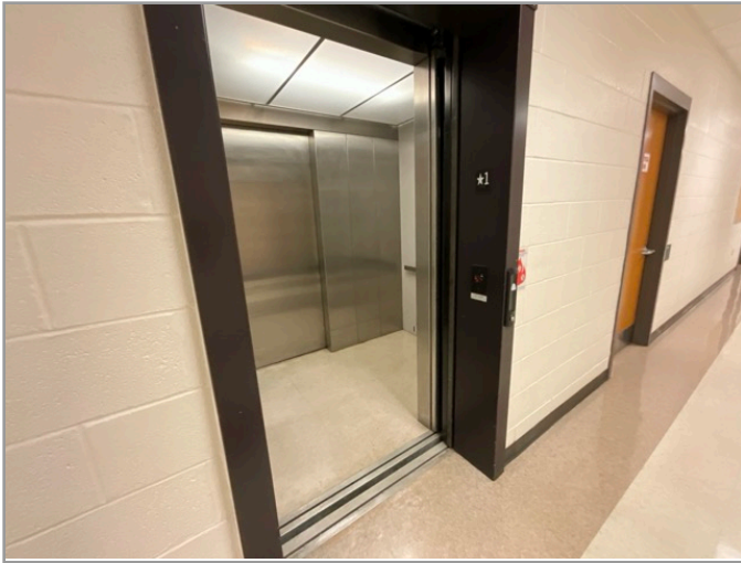
LOBBY LOOKING AT CABS (WITH DOORS OPEN)
