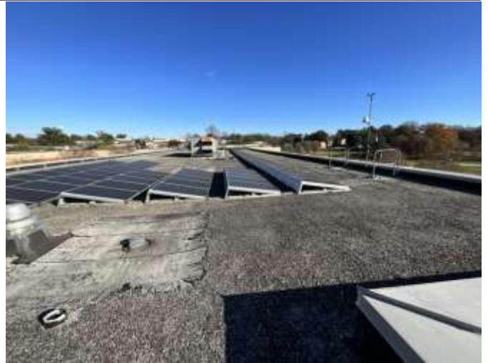
8 - PRIMARY ROOF OVERVIEW
