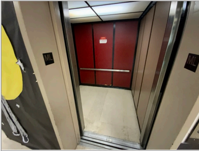
LOBBY LOOKING AT CABS
